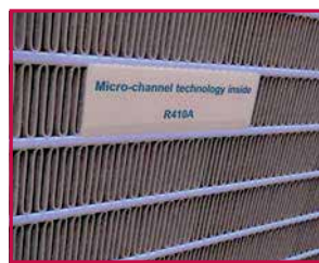
Aluminium micro channel heat exchanger
